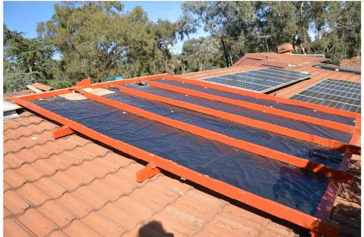
has a fan and the air is then distributed within the house. I am using an Arduino microprocessor that costs around \$30 to control it. Each duct has a temperature sensor and when 30 degrees is reached, the fan is turned on.
