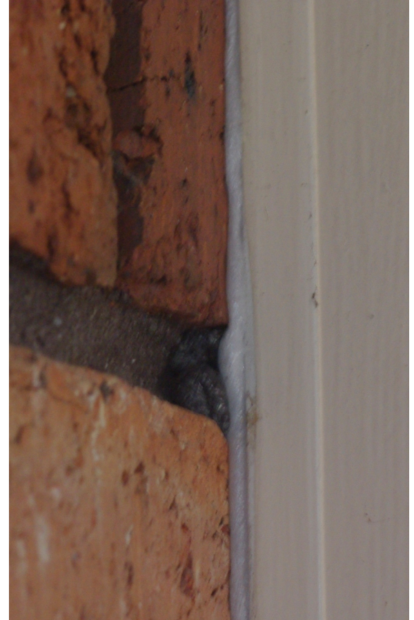
Filling the gaps
